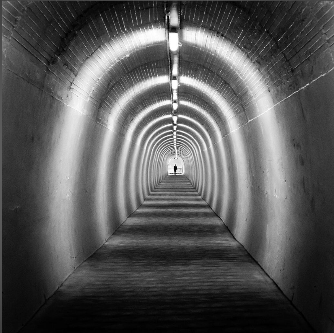
28 NZ-Durie Hill Tunnel
