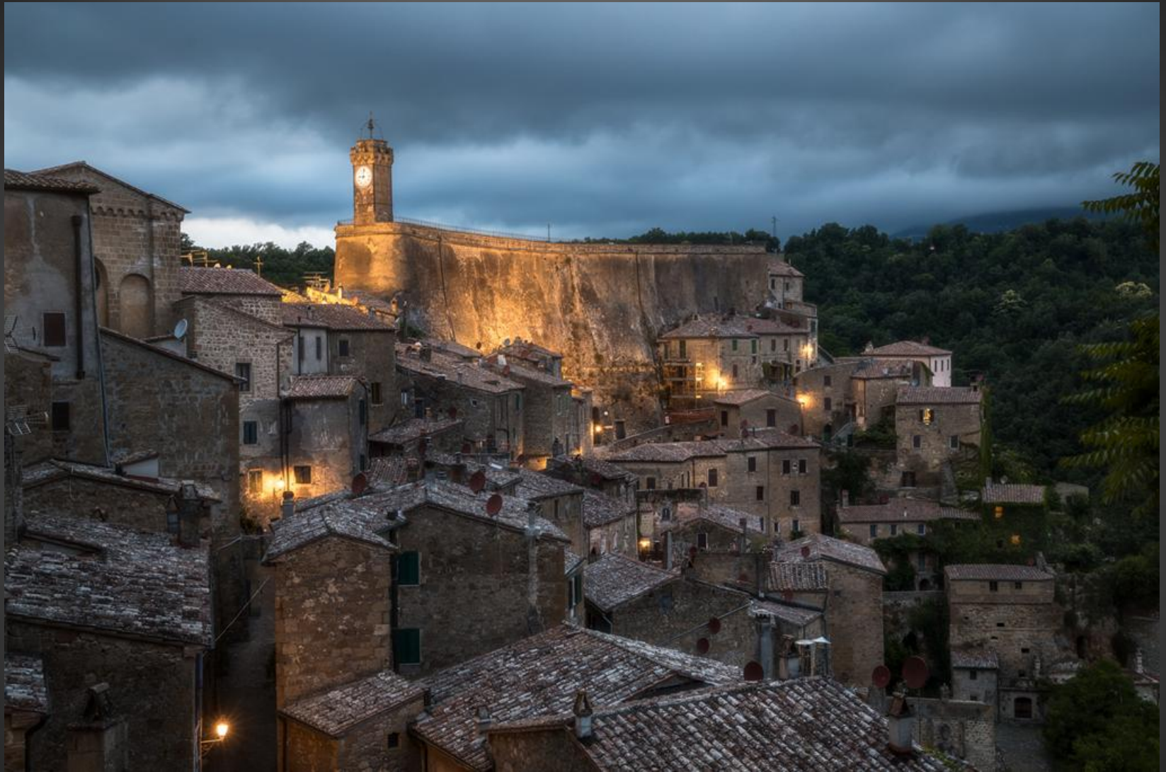
22 IT-The Roofs of Sorano
